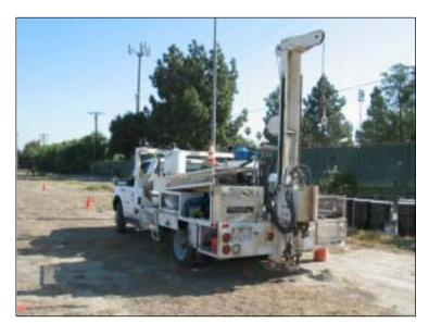
New air sparge wells were installed along the facility's eastern boundary in April 2007.
